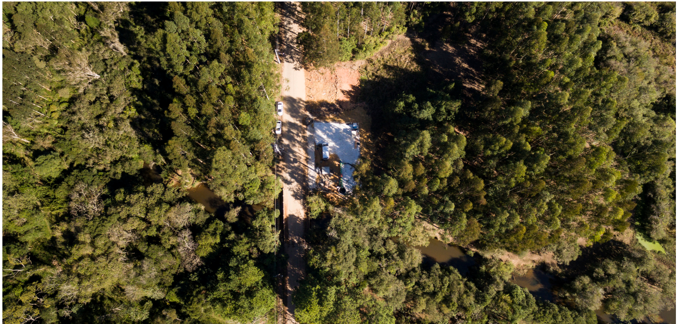
Rio Pequeno Emergency Funding Work – Photographer: André Thiago Chaves Aguiar
