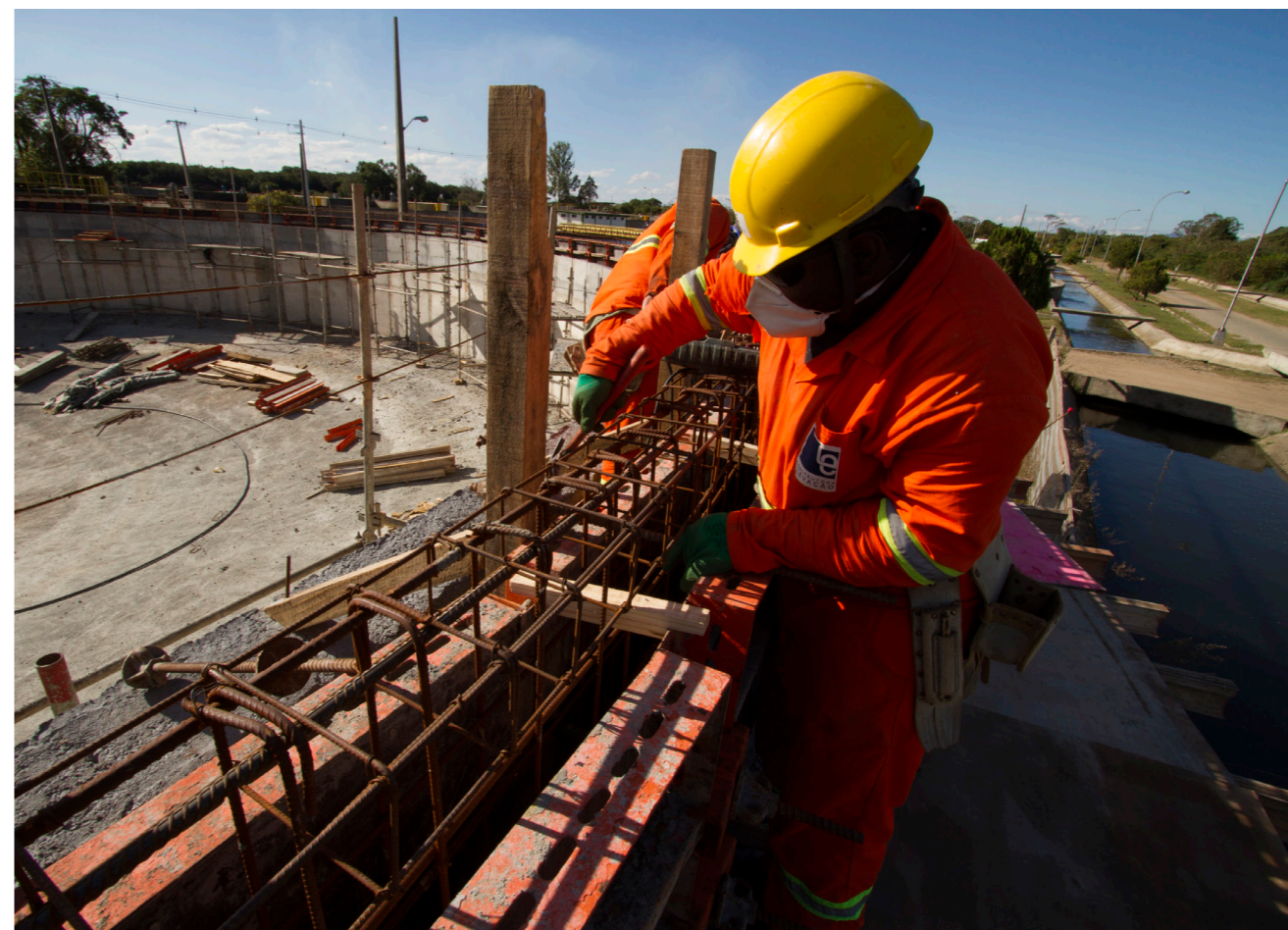
Work ETE Belém - Photographer: André Thiago Chaves Aguiar
